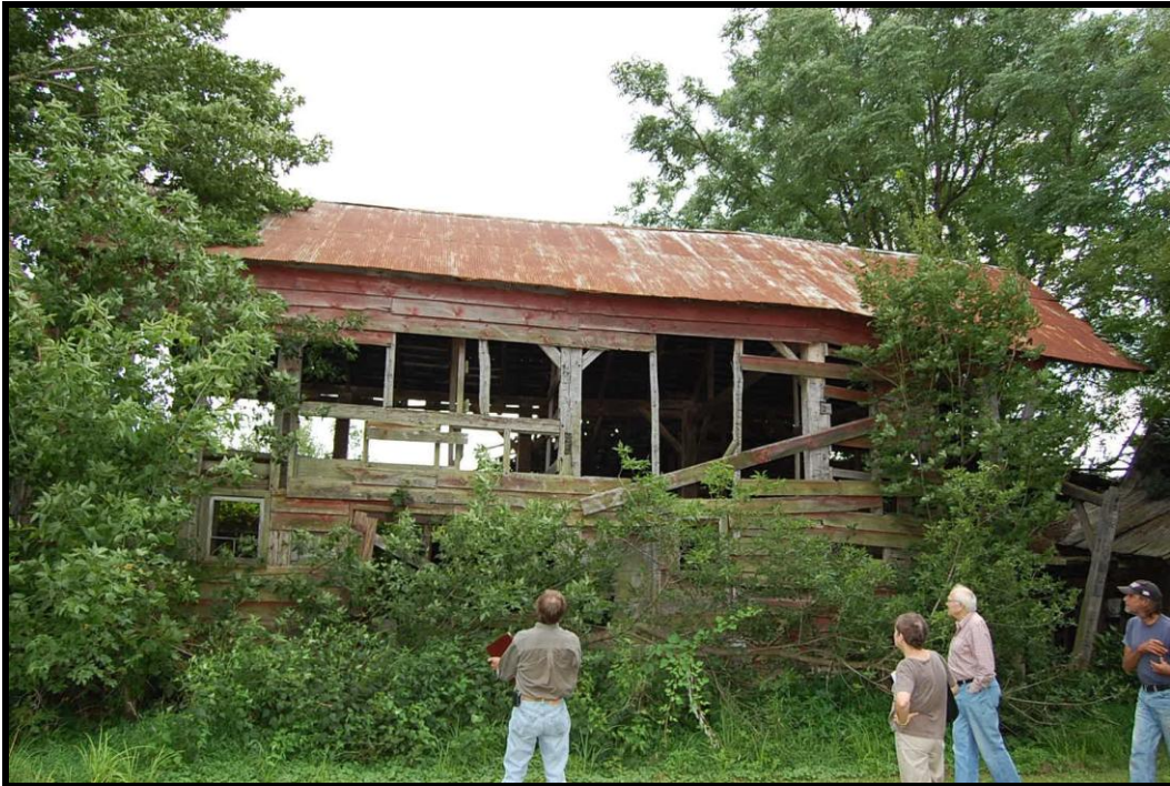
Figure 3. A more recent photograph of the Galloway Barn prior to dismantling.
